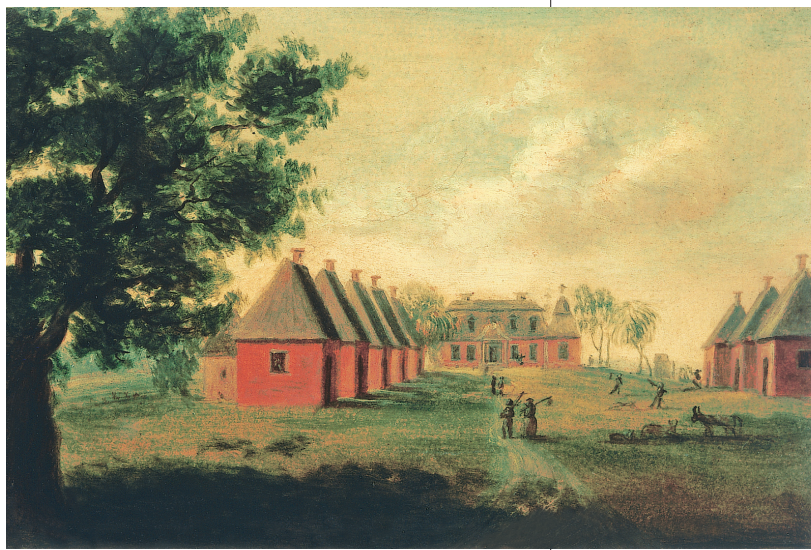
Above: Mulberry Plantation, a rice plantation in Moncks Corner, was established by Thomas Broughton in 1716. It is one of the oldest plantations in the country. This painting shows the slave quarters leading up to the plantation house in the center. The style of the slaves' huts reflects the style of their dwellings in Africa. Thomas Broughton later served as a royal governor of South Carolina.
